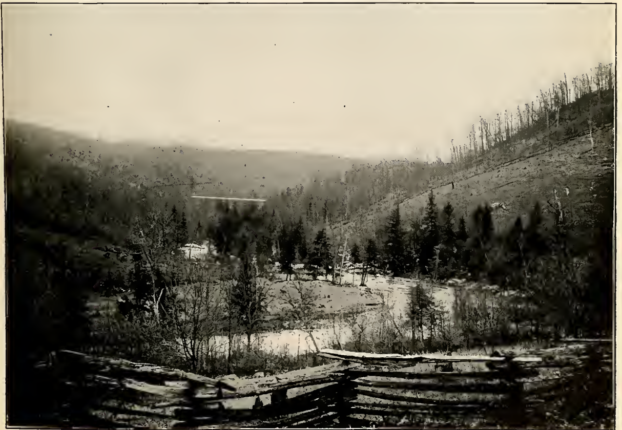
SANDY CREEK, W. VA., DECEMBER, 1910. View down stream, showing crest of proposed dam.
